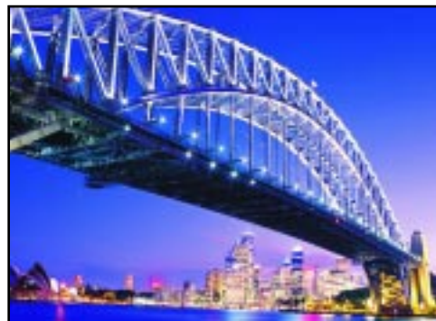
Bridge and Building Monitoring
